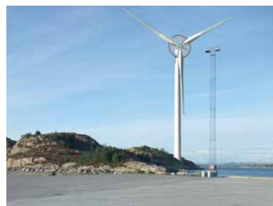
In 2010, Sway received support to build and test a self-developed wind turbine in Naturgas-sparken in Øygarden in Hordaland. The wind turbine will be the world's largest, with an installed capacity of 10 MW and a rotor diameter of 145 metres. Illustration: SWAY.
