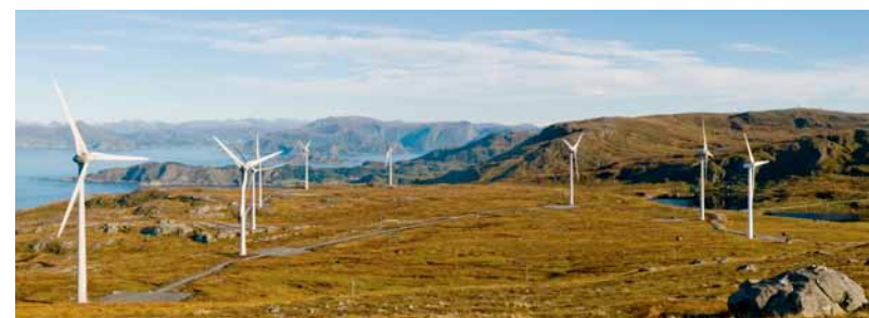
Mehuken II wind power plant was officially opened on 29 October. Overall, Mehuken I and Mehuken II generate approximately 65 GWh, which is equivalent to the annual end-use of 3 000 households. Photo: Einar Berg.
